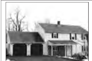
BRISTOL-THIS HOUSE has been totally remodeled in 1989, 3 BRs, 2.5 baths, eat-in kitchen, MBR w/full bath, nice open floor plan on 1 st floor. A lot of house for the money. ASKING $199,900.
